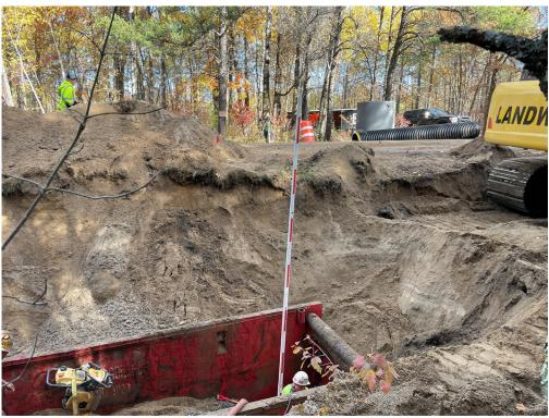
Photo #9: Measuring pipe elevation - Oct 20, 2023, 11:27 AM
