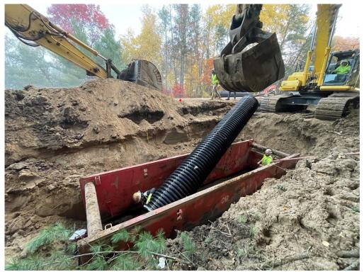
Photo #7: Installing first section of gravity flow pipe for the day - Oct 20, 2023, 7:55 AM
